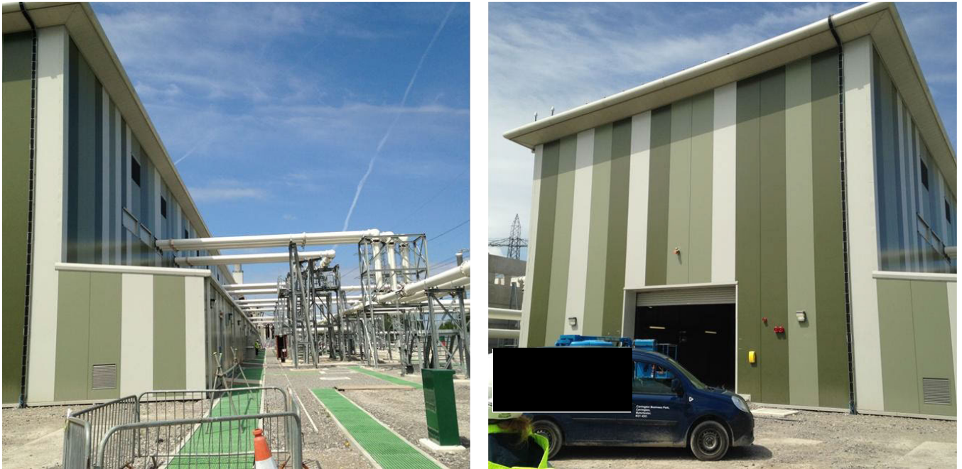
Image 3.6 and 3.7 National Grid Deeside Centre for Innovation 400 kV Substation (Source: National Grid)
