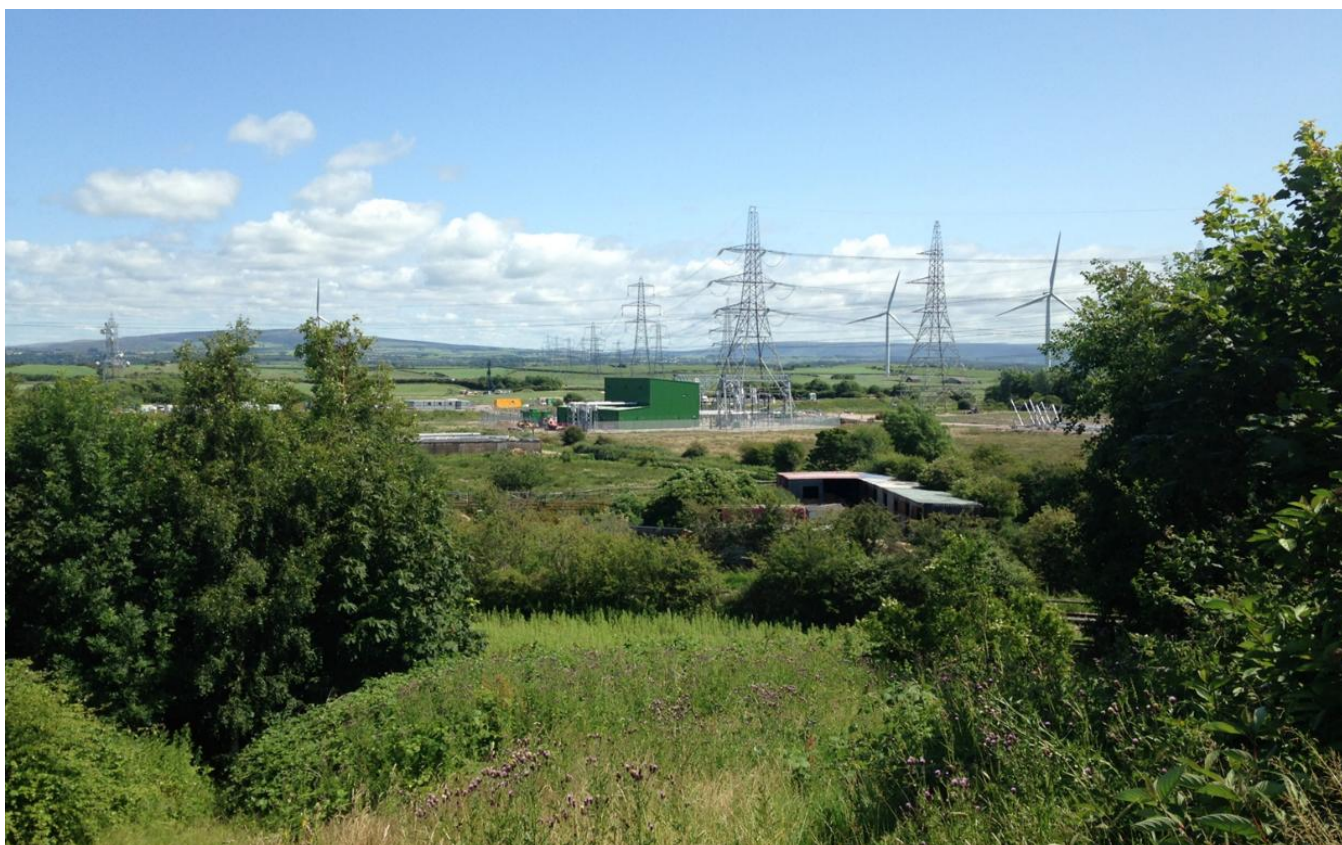
Image 3.5 Existing Middleton 400 kV Substation (Source: National Grid)
