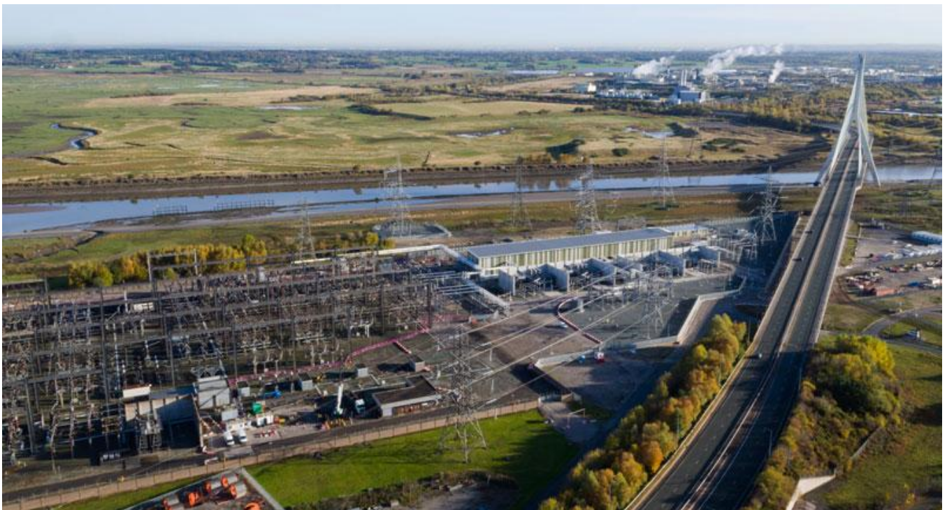
Image 3.3 Existing Connah's Quay 400 kV Substation in colour cladding (Source: National Grid)
